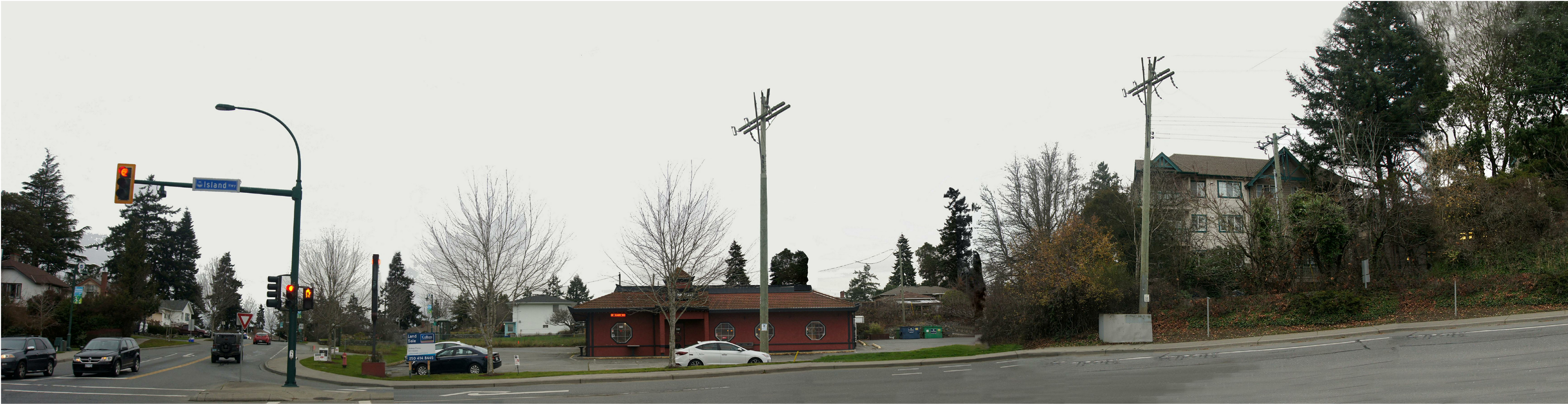
EXISTING STREET SCAPE ALONG ISLAND HWY
